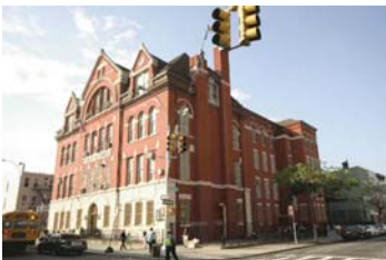
Fig. 43: Grand Street Settlement Day Care Center (Photo by Keenan Hughes)
