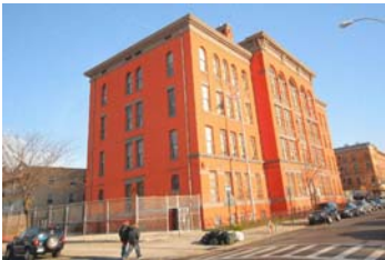
Fig. 42: Grand Street Settlement Day Care Center (Photo by Keenan Hughes)
