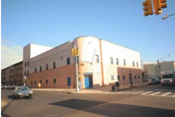
Fig. 33: Grand Street Settlement Day Care Center (Photo by Keenan Hughes)
