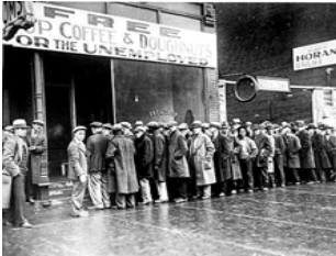
Fig. 15: Blows to industries: Depression (Source: www.hugosuboarchitects.com )
