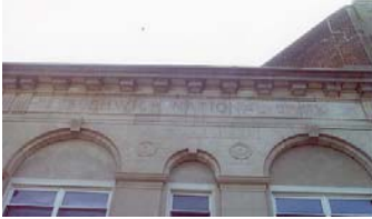
Fig. 53: Bushwick National Bank (Source: www.forgotten-ny.com )
