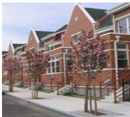
Fig. 21: New investments: Rheingold Site Redevelopment (Source: www.nyhomes.org )
