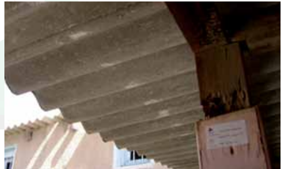
Detail of cement roof sheeting containing white asbestos
