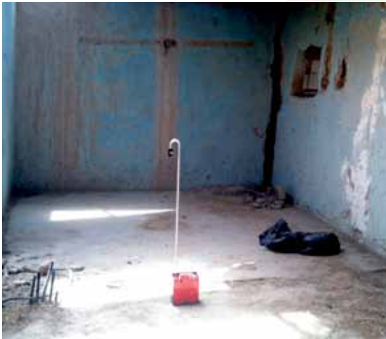
Monitoring the asbestos particles in the air around the site
