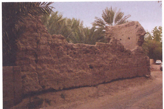
{ 15/1/2010, The state of the building before the emergency conservation intervention }
