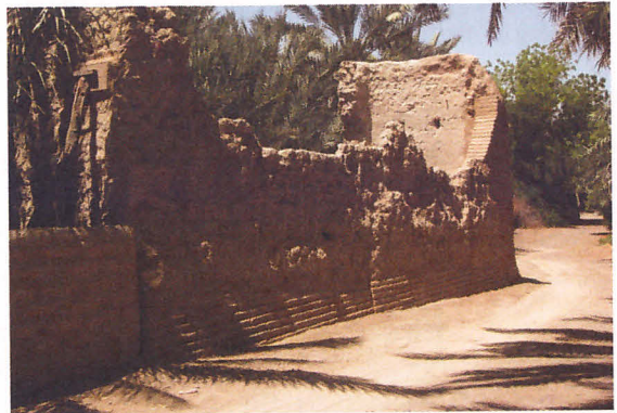
{ 5/5/2010, The building after completing the emergency conservation intervention }
